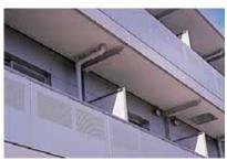
Blind panel under balcony handrail, partially perforated panels, Japan
